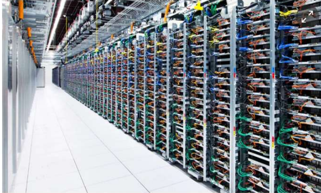
Inside Google's data centre in Mayes County, Oklahoma. The firm's carbon footprint was equivalent to more than 1.7m tonnes of carbon dioxide in 2013. Photograph: Google/Rex
